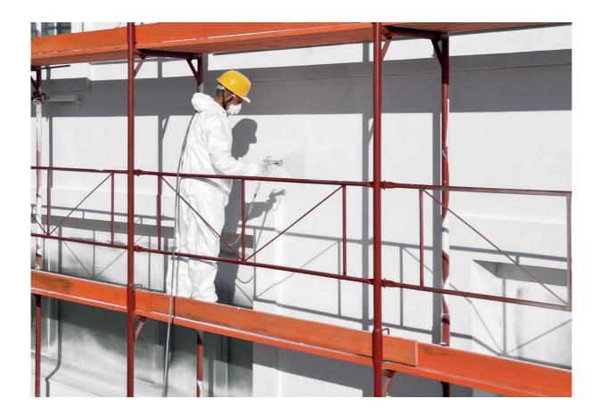
When spraying, always make sure that the spray gun is held perpendicular to the surface to be sprayed, at the distance defined by the nozzle, and that the spraying equipment maintains the operating pressure and spray profile without disturbance, as this is the only way to achieve a proper spray pattern. The spray radius must be uniform. If streaks appear in the spreading radius, the spreading pressure is too low. In this case, the pressure should be increased.
