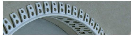
The edges of curved plasterboard surfaces can be made into unbreakable edges by incorporating bendable edge protectors.
